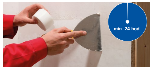
Picture No. 8: Covering of the edges.
