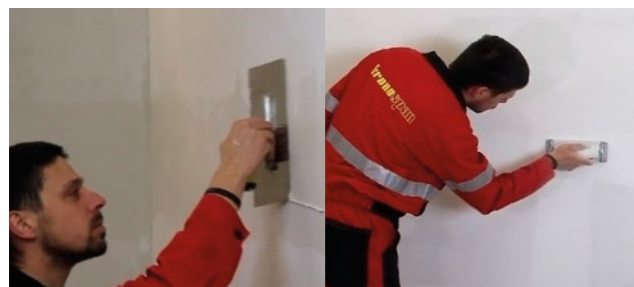
Picture No. 9: Covering of the edges.
